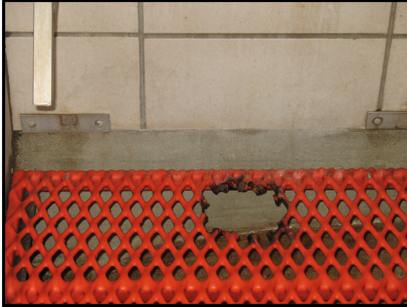
Drain holes have rough edges and are not covered. Staff reported that dogs have gotten trapped and had to be killed in kennel to be extricated.
